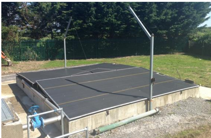
Figure 1: Sludge Drying Beds at Twomileborris WWTP.
