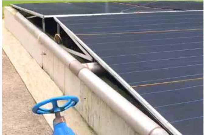
Two units in parallel in a 650PE WWTP
